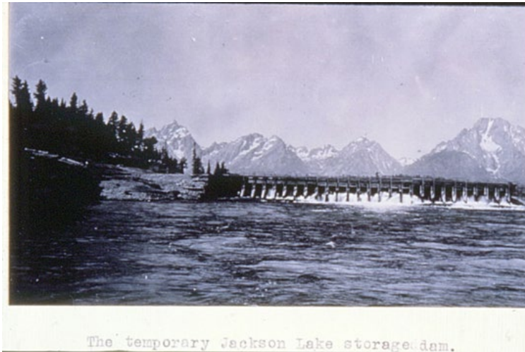
The temporary Jackson Lake storage dam.
